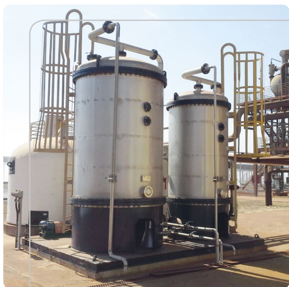
Usina Colorado - SP - 50m 3 h
