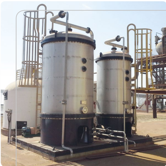
Usina Colorado - SP - 50m 3 h
