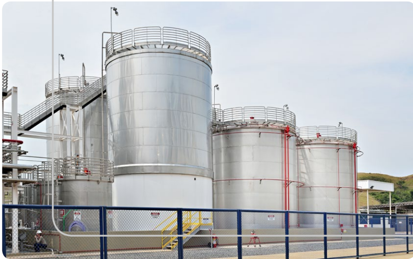
Beverages - Storage Tank - Ambev Pirai - RJ
